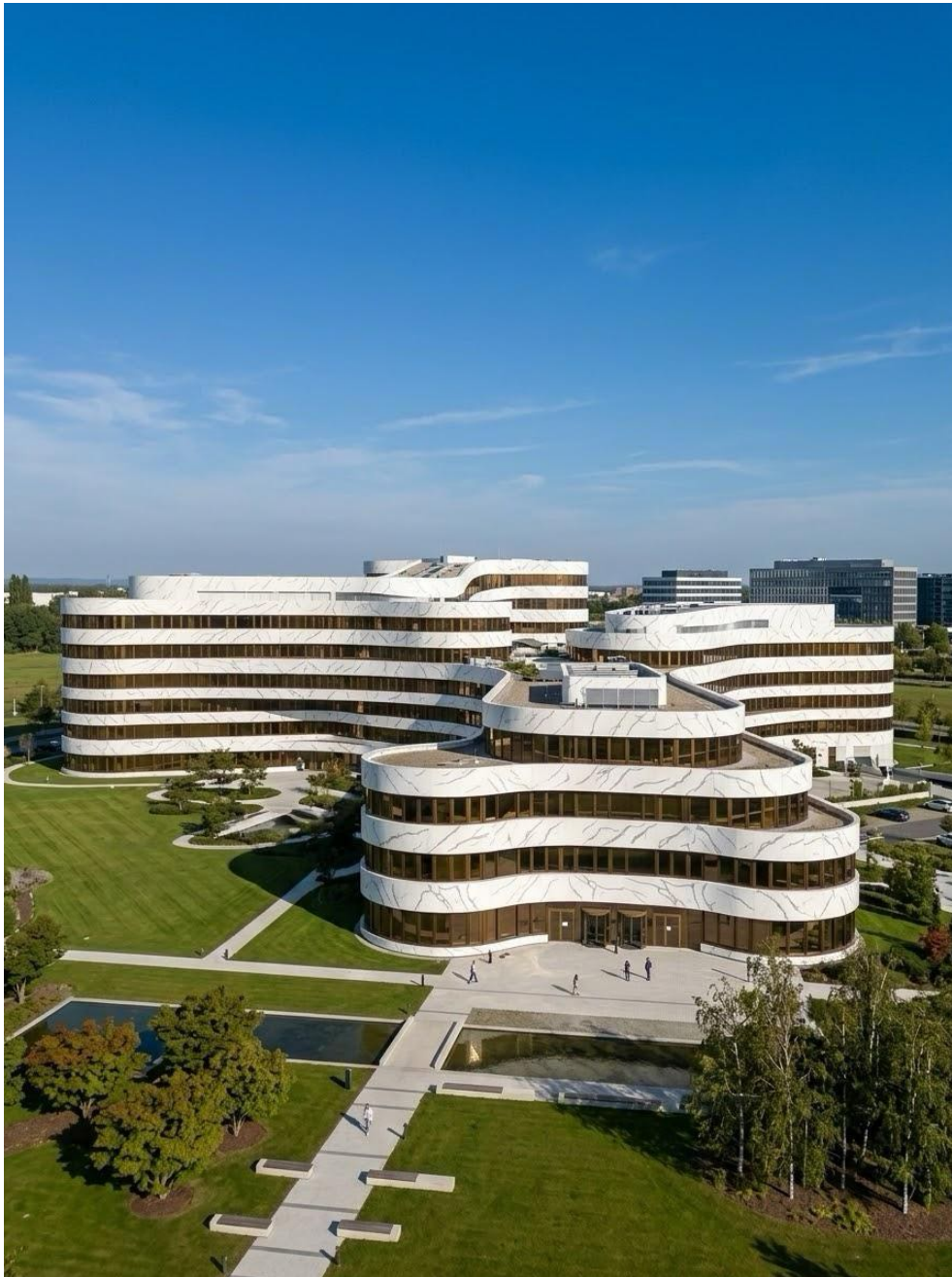
Advanced ventilated facade application using MaryFass Acrylic Solid Surface
